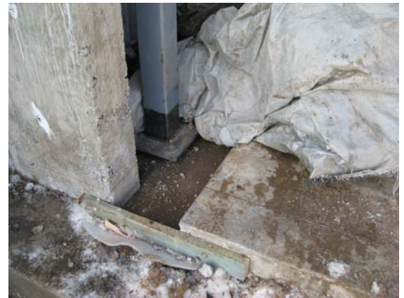
FIGURE 4 – COLUMN BASE PLATE BLOCK-OUT
