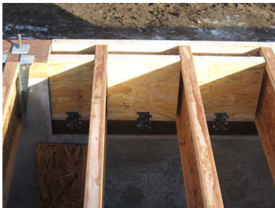
FIGURE 5 – JOIST AND RIM BOARDS INSTALLED PER PLANS
