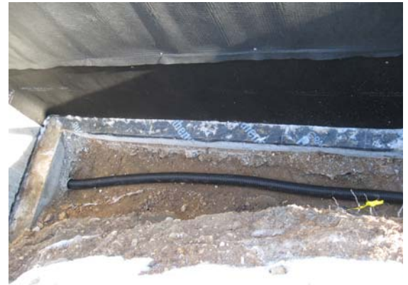
FIGURE 3 – DRAINAGE AND STEM WALL INSULATION
