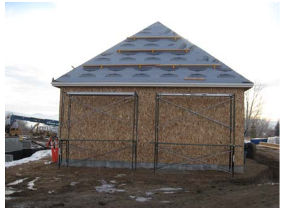
FIGURE 1 – COMPLETED UPPER GARAGE
