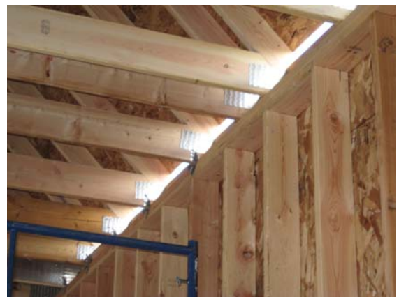
FIGURE 2 – HURRICANE TIES INSTALLED ON THE INTERIOR OF STRUCTURE.
